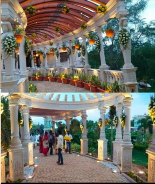
Sandstone Elevation Resort work
