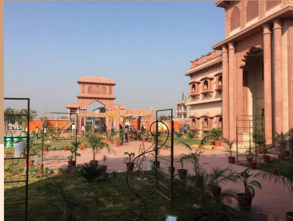
Sandstone Elevation Resort work
