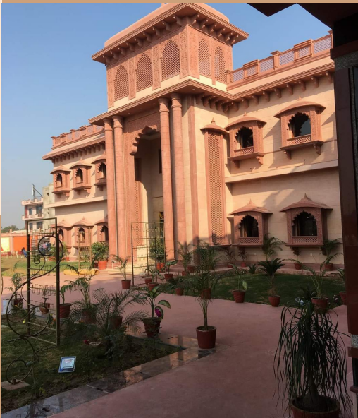
Elevation Sandstone Work
