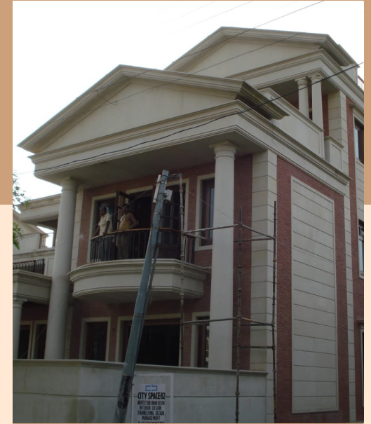
Sandstone Building Elevation
